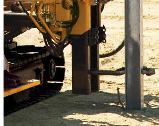
It might not seem like much, but when multiplied by the number of posts driven during the course of a solar farm job, it's precious time saved by tapping into 3D machine control to augment pile driving machines. Seconds matter, and they add up. It didn't take long for IEA, an infrastructure construction company with specialized energy and
